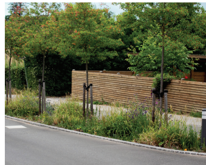
Green stormwater street - Kong Hans Alle (Copenhagen, Denmark)
