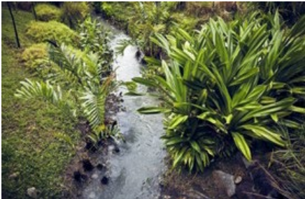
Rainwater harvesting for cooling tower water
