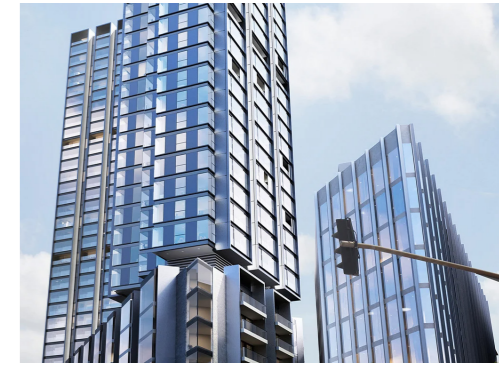
250 City Road (38 Storey residential) Credits: Foster + Partners
