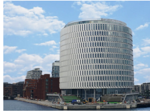
Redmolen spidsen, Denmark
